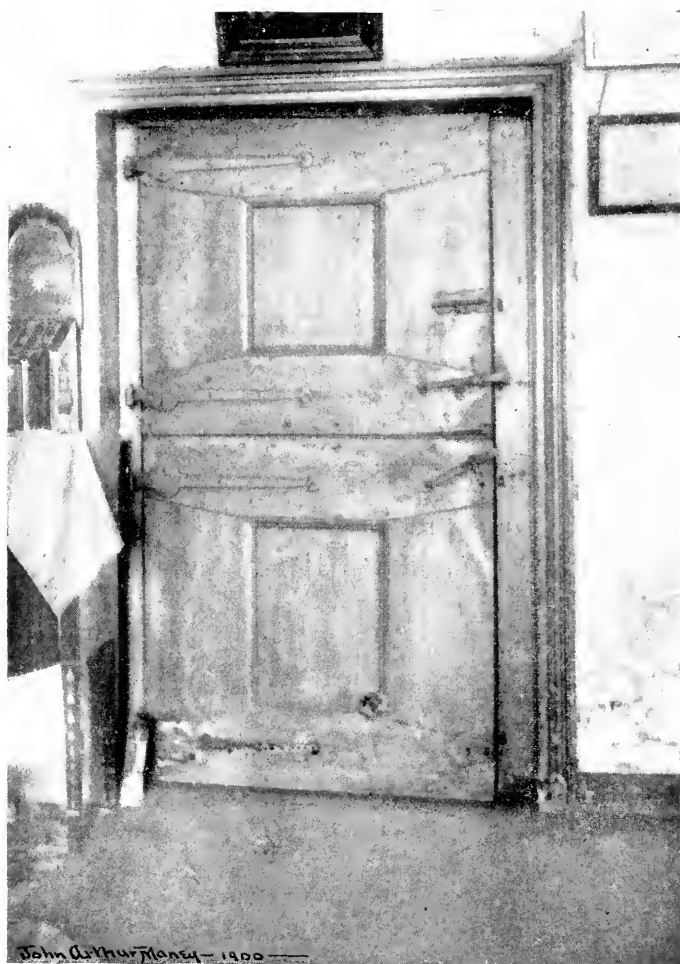
DOOR IN THE GLEN-SANDERS HOUSE
