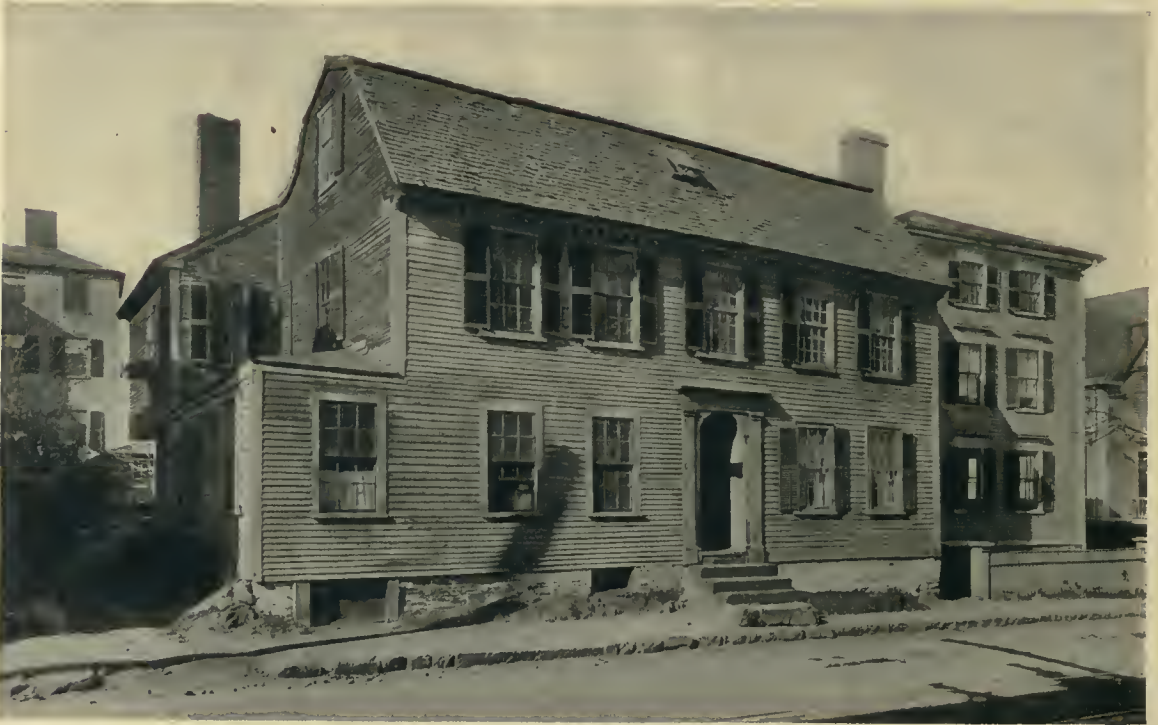
A HOUSE ON STATE STREET, MARBLEHEAD, MASSACHUSETTS.
