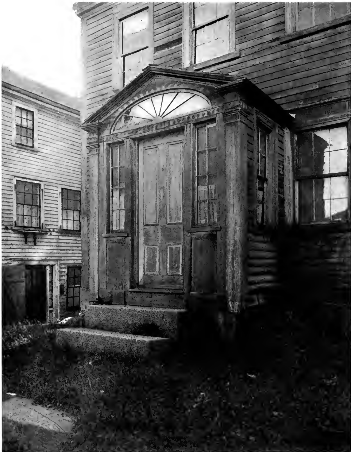
HOUSE IN LOOKOUT COURT, MARBLEHEAD, MASSACHUSETTS. Detail of Entrance. The elliptical fan-light and reeded pilasters give to this very old house a distinct architectural character.
