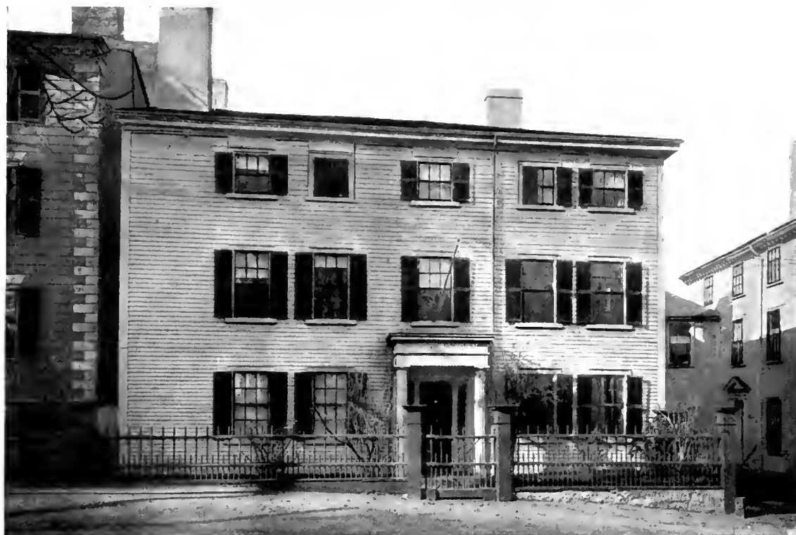
HOUSE ON WASHINGTON STREET, MARBLEHEAD, MASSACHUSETTS.
