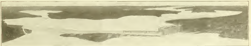
Source of additional power for Winnipeg Electric Railway Company.—The Great Falls development on Winnipeg River—Capacity 168,000 h.p.
