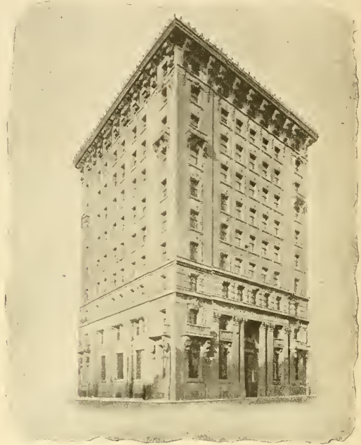
BANK OF NOVA SCOTIA'S NEW PREMISES AT 263 ST. JAMES STREET, MONTREAL
