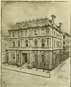
Head Office Building, Montreal
