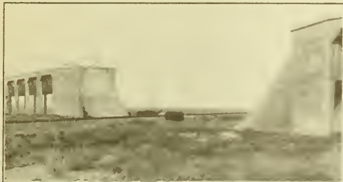
BROOKS AQUEDUCT—SHOWING INVERTED SYPHON UNDER MAIN LINE OF THE C.P.R.
