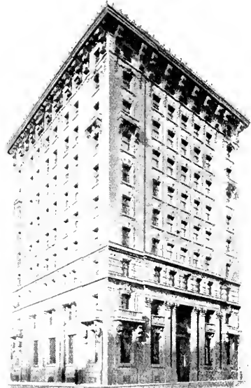
BANK OF NOVA SCOTIA'S NEW PREMISES AT 263 ST. JAMES STREET, MONTREAL
