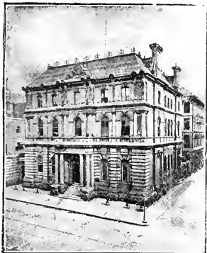
Head Office Building, Montreal
