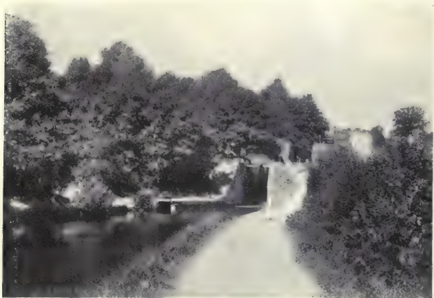
The Brecon and Newport Canal, near Newport
