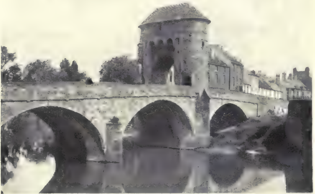
Bridge over the Monnow at Monmouth
