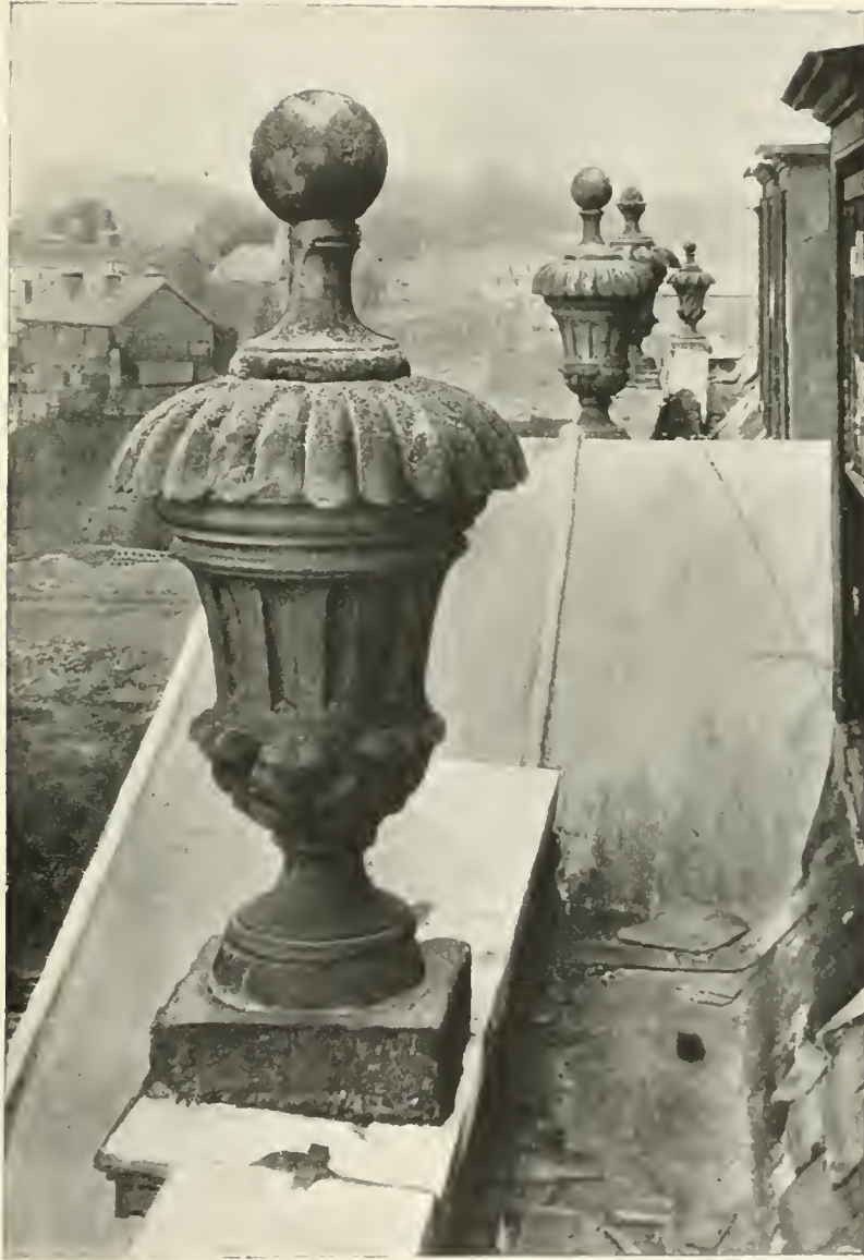
VASES ON PARAPET OF ROOF, ENTRANCE FRONT.
