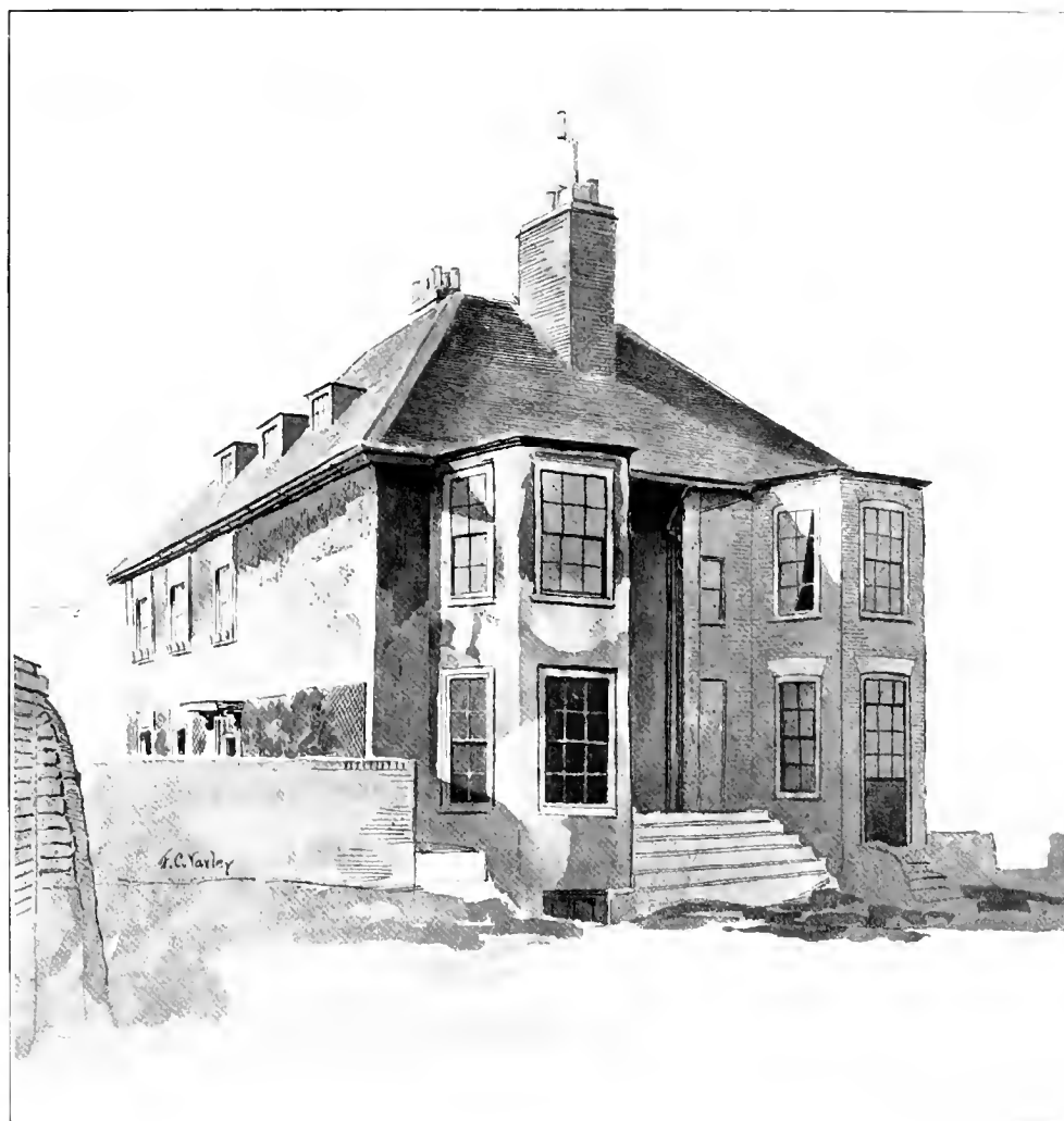
VIEW FROM SOUTH-WEST.
