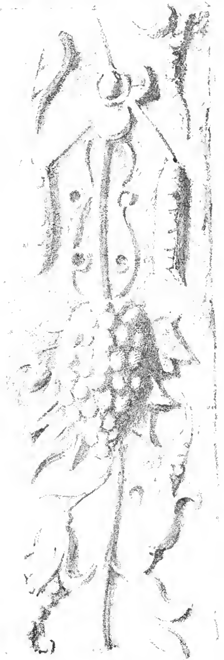
ORNAMENT ON CEILING WITH N.W. SIDE DROPPING FLOOR
