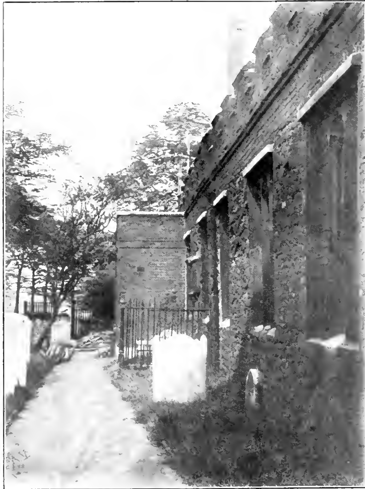
The North Aisle Wall and Old Vestry.
