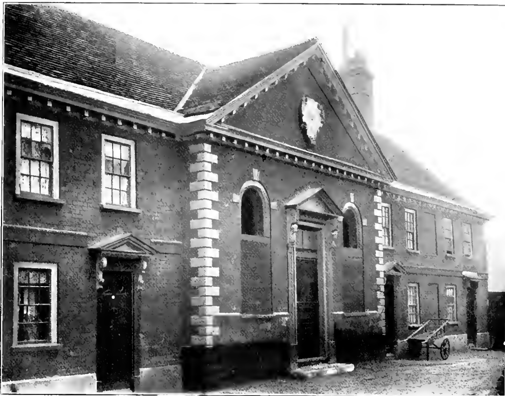
VIEW FROM NORTH-EAST.
