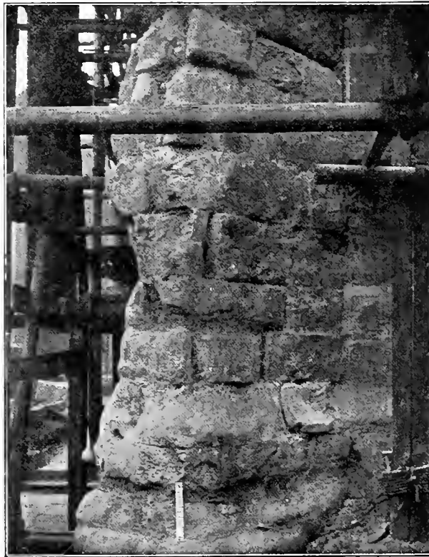
The South-West Buttress of the Tower.
