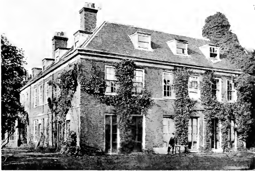
SOUTHERN AND WESTERN FRONTS.
