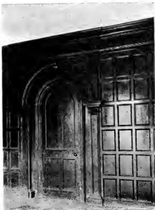
PANELLING AND DOORWAY.
