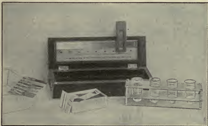
Fig. 18.—Kienboeck's Quantitimeter. (By courtesy of the Schedel-Western X-ray Coil Co.)
