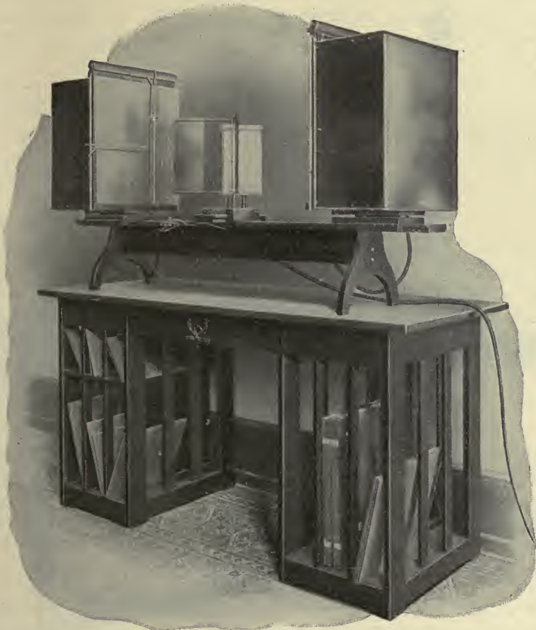
Fig. 27.—The Wheatstone Stereoscope. (By courtesy of the Röntgen Mfg. Co.)
