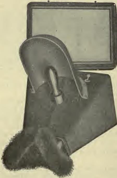
Fig. 21.—Lead-protected Röntgenoscope. (By courtesy of the Scheidel-Western X-ray Coll Co.).
