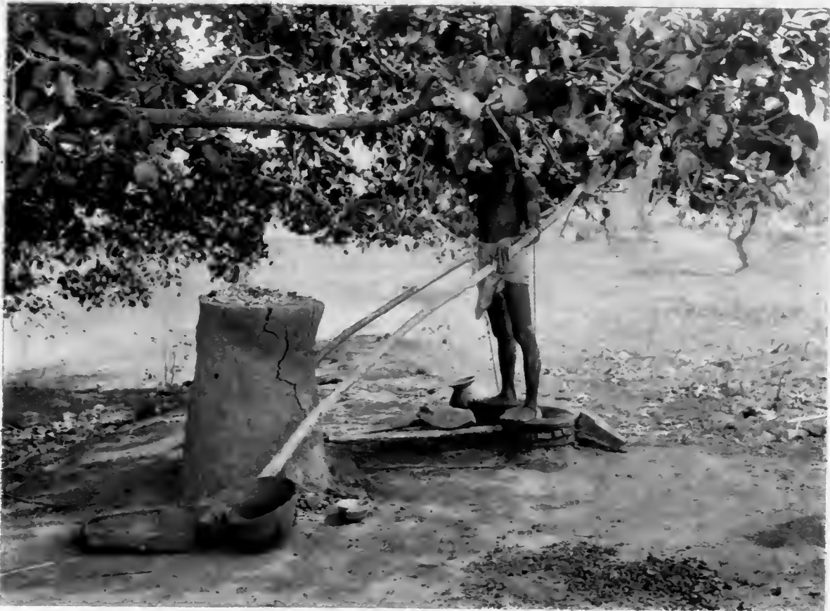
FIG. 1. IRON-SMELTING IN THE SONTHAL PARGANAS.
