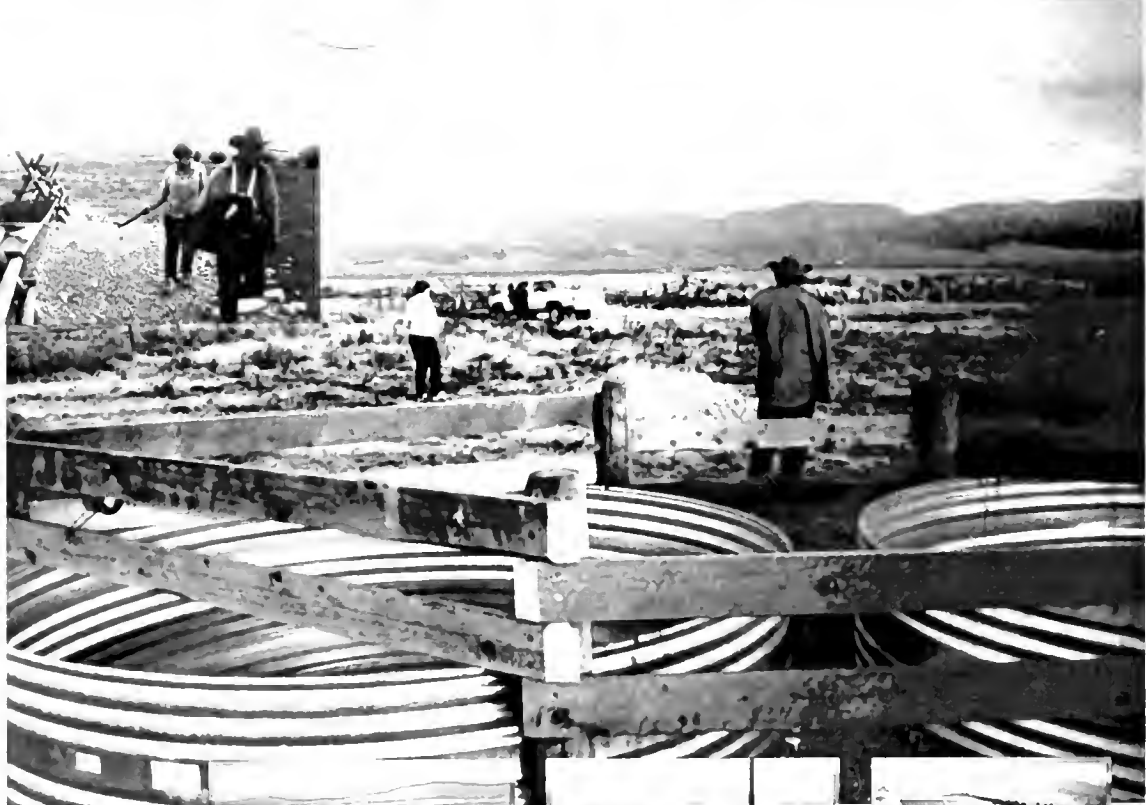
Large capacity stockwater tank
