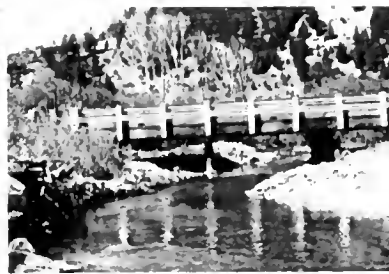
After construction—note that the willow has been removed and placed on the side of the channel. Note also how the channel is no longer endangering the bridge
