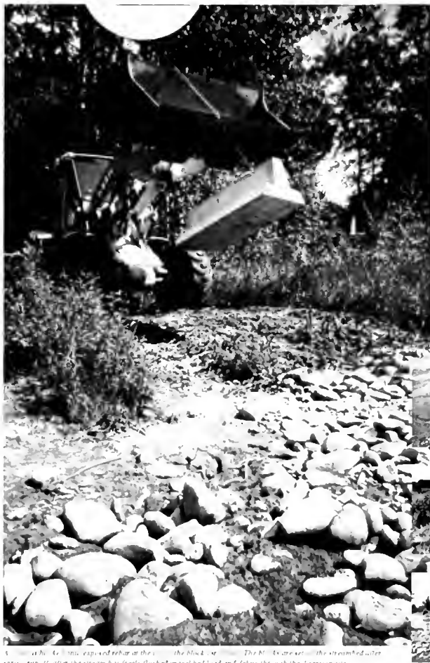
Figure 1. The 1997 diversion structure on the Nichols-Burrell Ditch. The blocks were placed in the streambed after the stream has been flushed of gravel and debris through the diversion site.
