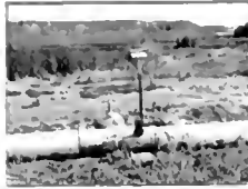
Irrigation sarge valve
