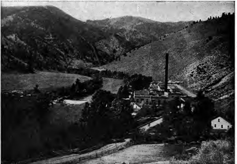
BUTTE PUMPING PLANT
