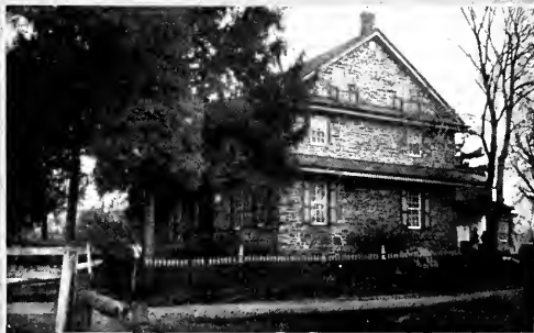
HIGH SCHOOL, POTTSTOWN—NOBLE STREET SCHOOL, NORRIS-TOWN—WASHINGTON'S HEADQUARTERS, NEAR CENTER POINT
