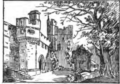
Belted Will's Tower, Naworth.
