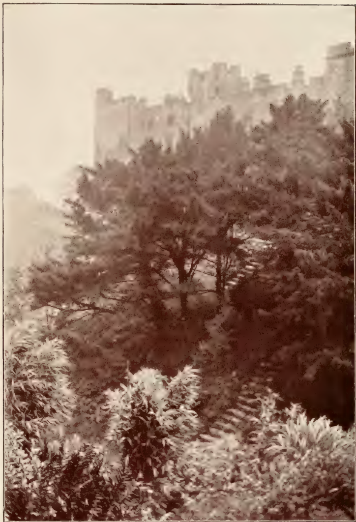
MUNCASTER CASTLE FROM THE ENTRANCE TO THE TERRACE WALK.
