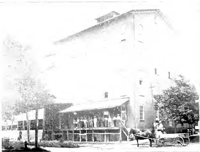
LOUGHRY MILL, the largest Mill In White County.
