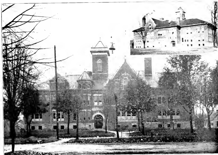
HIGH SCHOOL BUILDING, North and South View.
