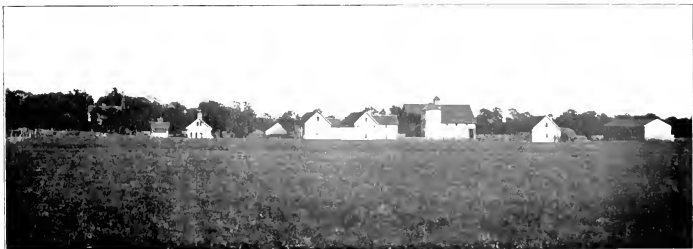
Buildings on A. A. McKain Dairy Farm, one mile south of Monticello.
