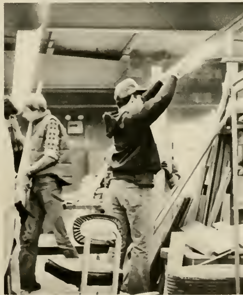
Jack Dever does some repair work on the PAC building for the organization.
