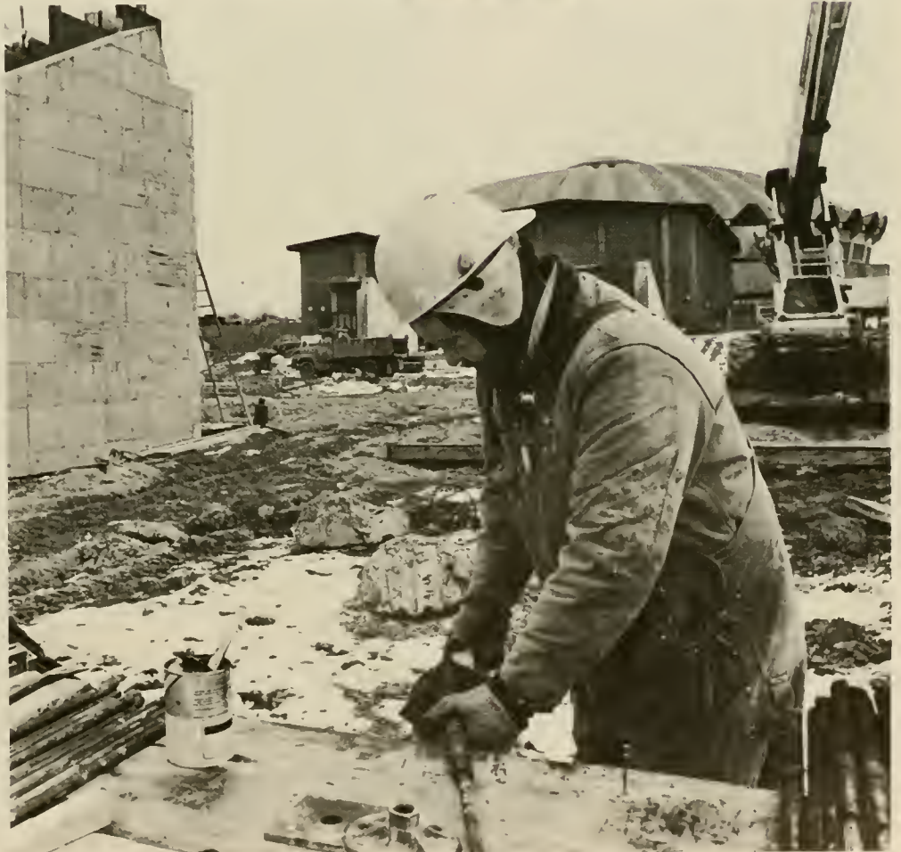
Stadium construction perseveres through a mild winter.
