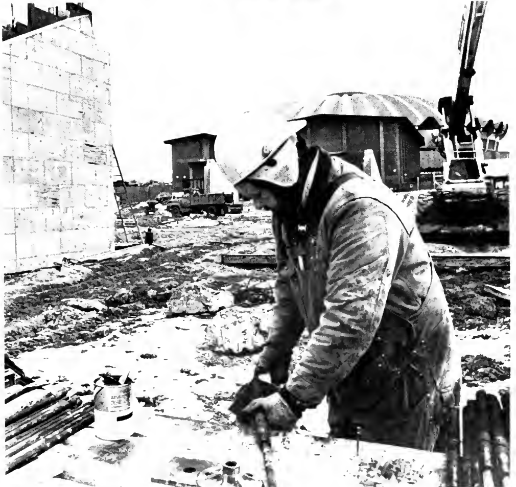
Stadium construction perseveres through a mild winter
