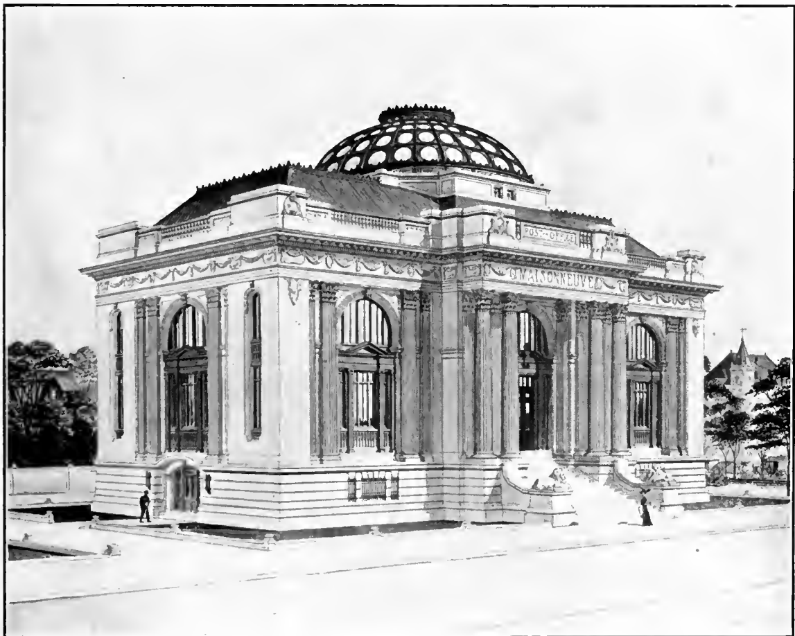
THE POST OFFICE UNDER CONSTRUCTION AT MAISONNEUVE.
