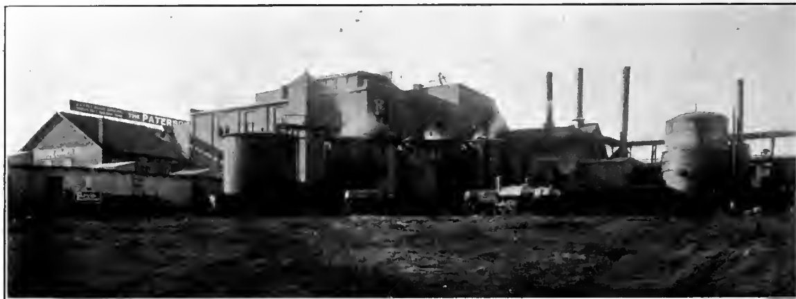
A PARTIAL VIEW OF THE WORKS OF THE PATERSON MANUFACTURING COMPANY, LIMITED.
