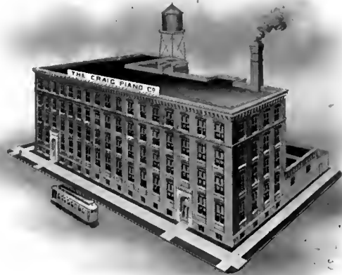
Craig Piano Co. Factory on St. Viateur Street.
