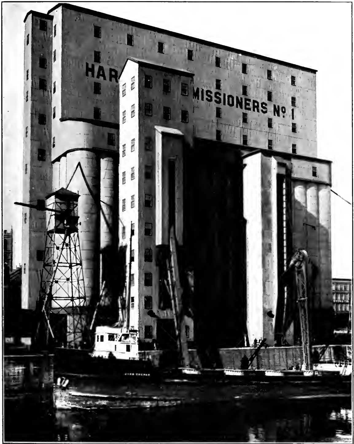
COMMISSIONERS ELEVATOR NO. 1, MONTREAL.
