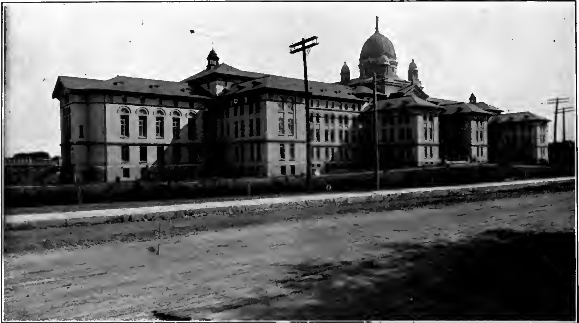
MOTHER HOUSE OF THE CONVENT OF THE CONGREGATION OF NOTRE DAME, Sherbrooke Street West, from which are directed a multiplicity of Montreal schools and colleges.
