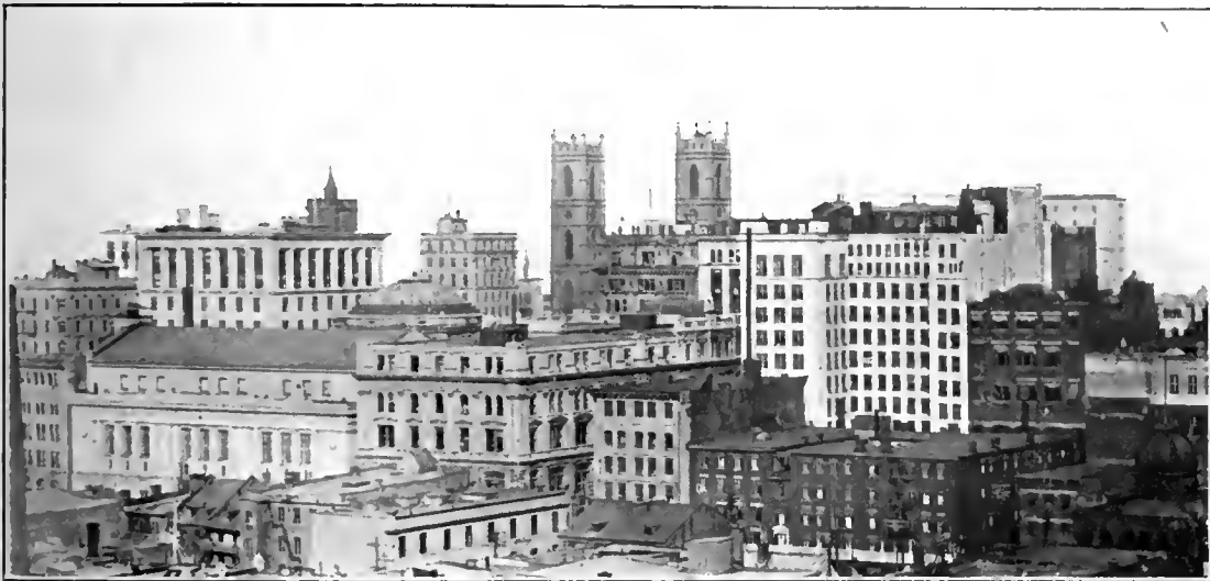
A section of the down town district of Montreal of to-day, which centres about the post office. The view is from the new Southam building on Bleury Street.
