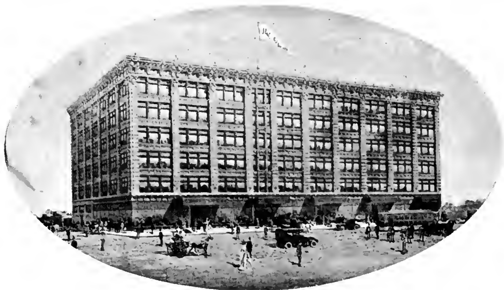
THE JACOBS BUILDING.
