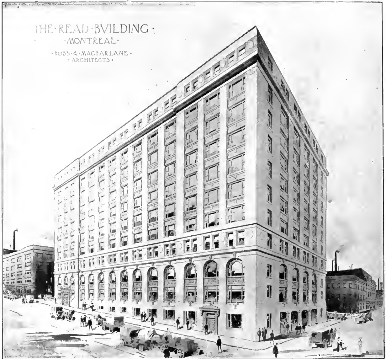
The Read Building, covering the entire block on Alexander, between Jurors and Laugachetiere Streets. One of the largest and most complete in the world.
