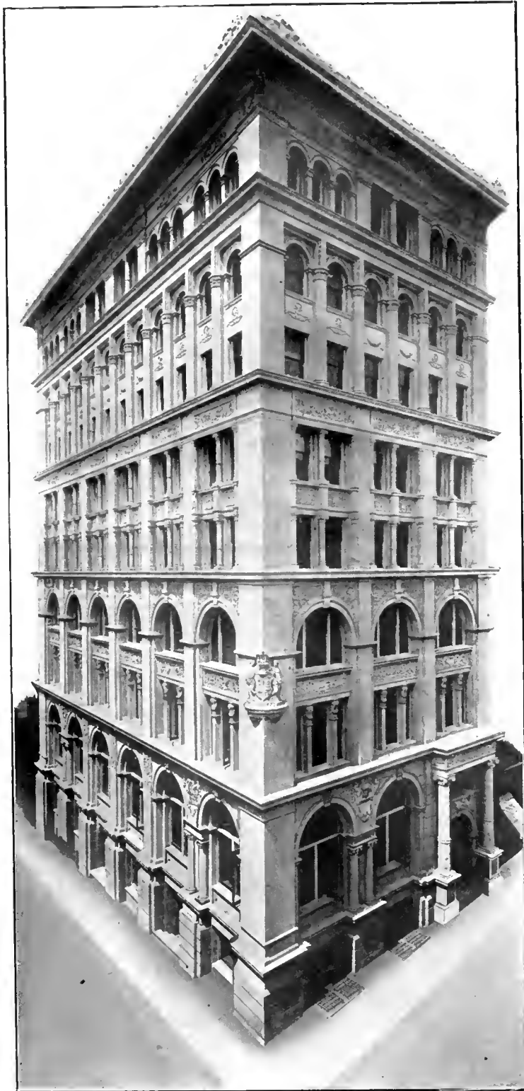
THE CANADA LIFE ASSURANCE COMPANY BUILDING AT MONTREAL.
