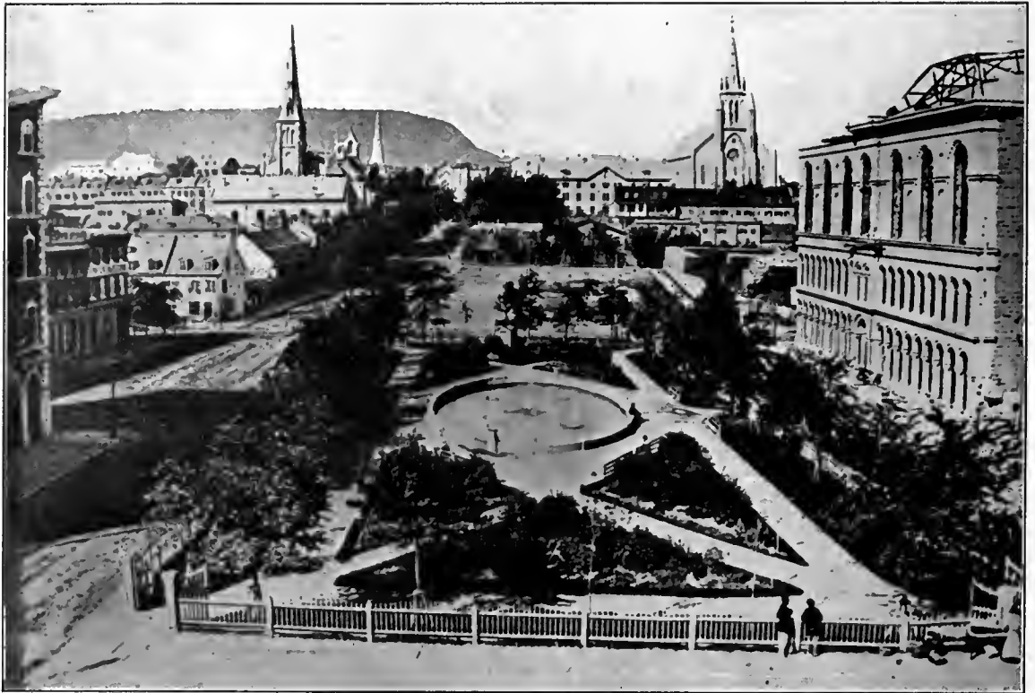
Victoria Square of fifty years ago. St. Patrick's Hall, in process of construction. Note the fence around the Square and the building at the extreme left standing squarely in the street.
