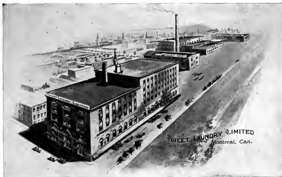
PLANT OF THE TOILET LAUNDRY CO., LIMITED, launderers, dyers and cleaners. Largest of the kind in Canada. Electrically equipped. 425 Richmond St., Montreal. Phone, Up 7640.
