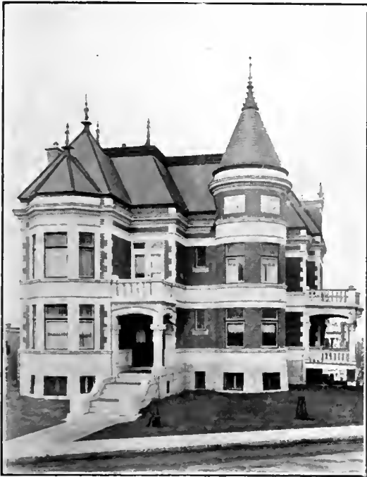
Handsome residence of Mr. Theo. Trudeau, at 191 St. Catherine Road, Outremont.
