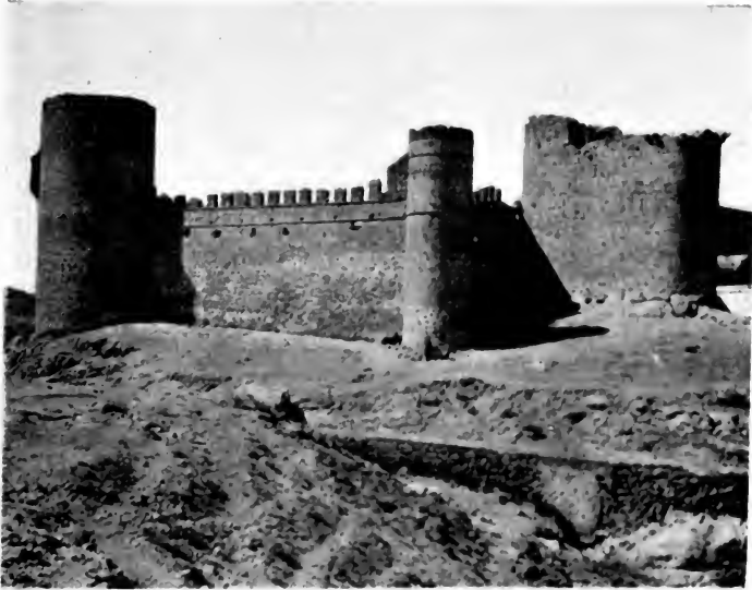
CASTLE OF ST. SERVANDO.
