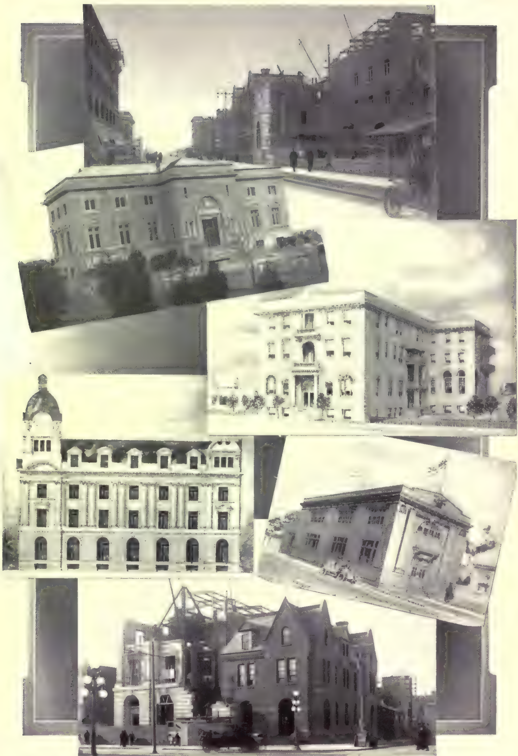
PUBLIC BUILDINGS UNDER CONSTRUCTION
