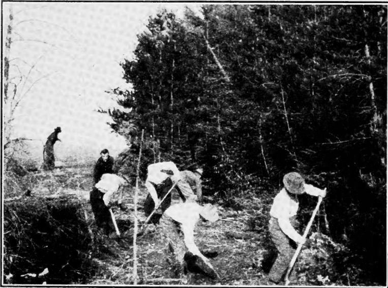
Fire Fighting Crew, Trenching ahead of a Fire
