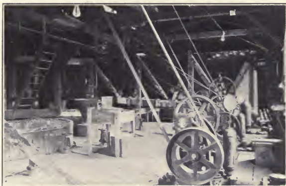
Fig. 40. PUMP ROOM, CYANIDE PLANT, MONTANA-TONOPAH MILL
