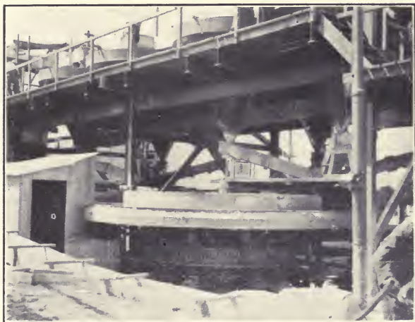
Fig. 71. CONTINUOUS SAND COLLECTOR
