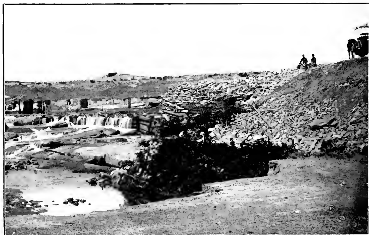
THE FIRST PERMANENT DAM ON THE LITTLE COLORADO AT ST. JOSEPH
