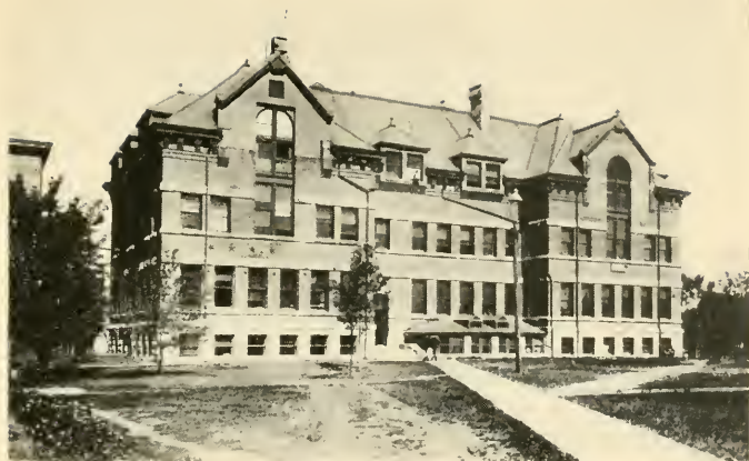
NEBRASKA HALL, THE RIGHT WING OF WHICH WAS USED FOR THE NEBRASKA STATE MUSEUM, WHERE THE MORRILL GEOLOGICAL COLLECTIONS WERE HOUSED UNTIL 1907.
