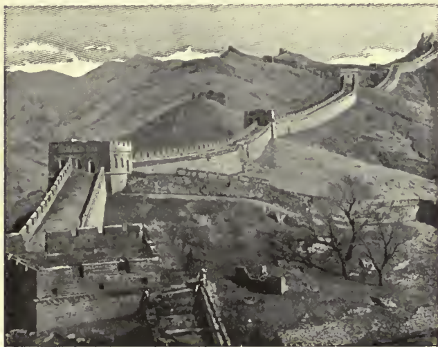
A part of the Great Wall of China.
