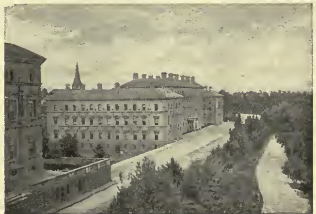
Government buildings, Melbourne.
