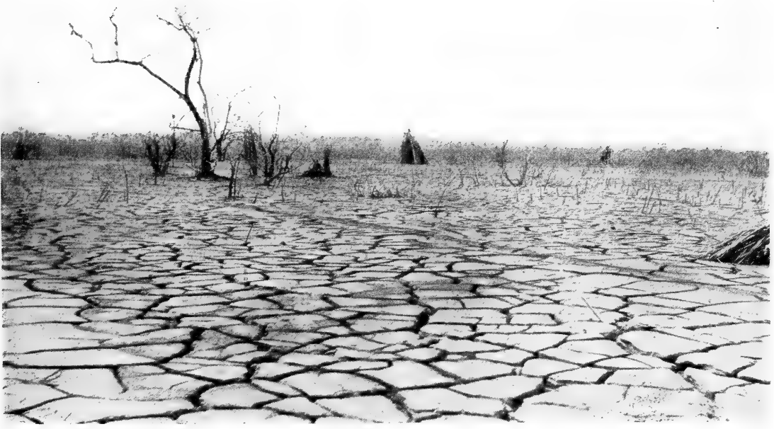
Cracks in a hydraulic fill
