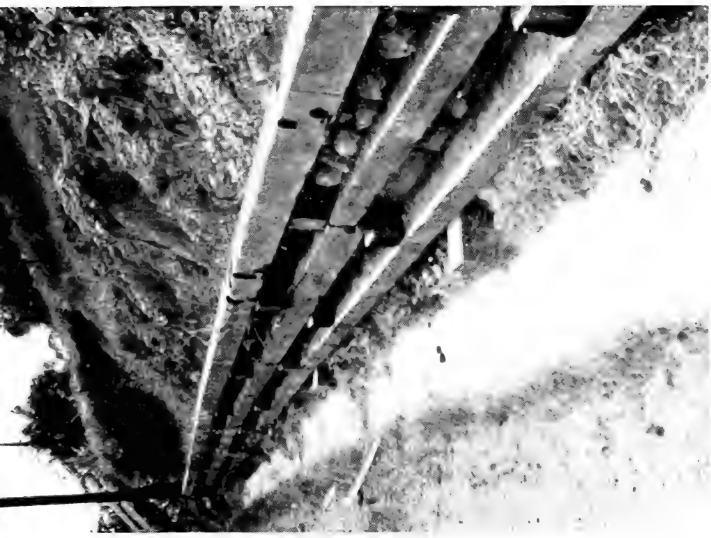
Reinforced thin concrete lining of a roadside ditch, and support of sliding toe of hill with
