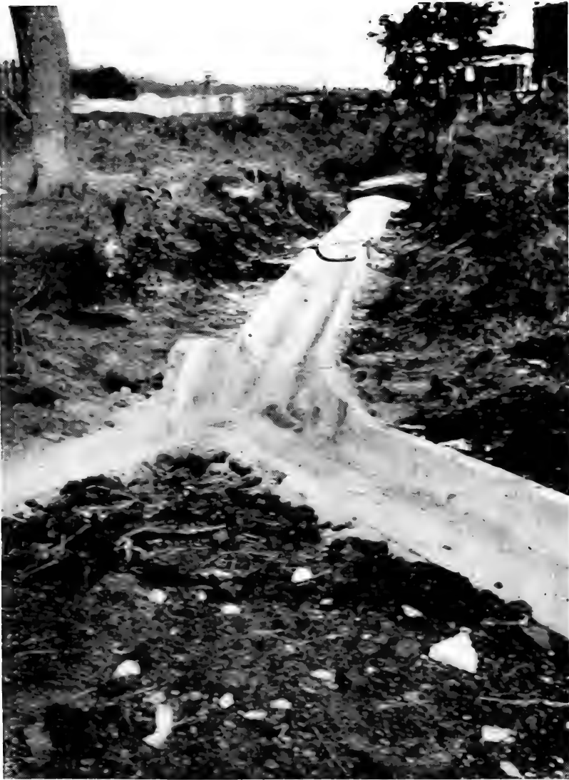
Junction of concrete ditches, showing splash wall to confine water within the ditch
