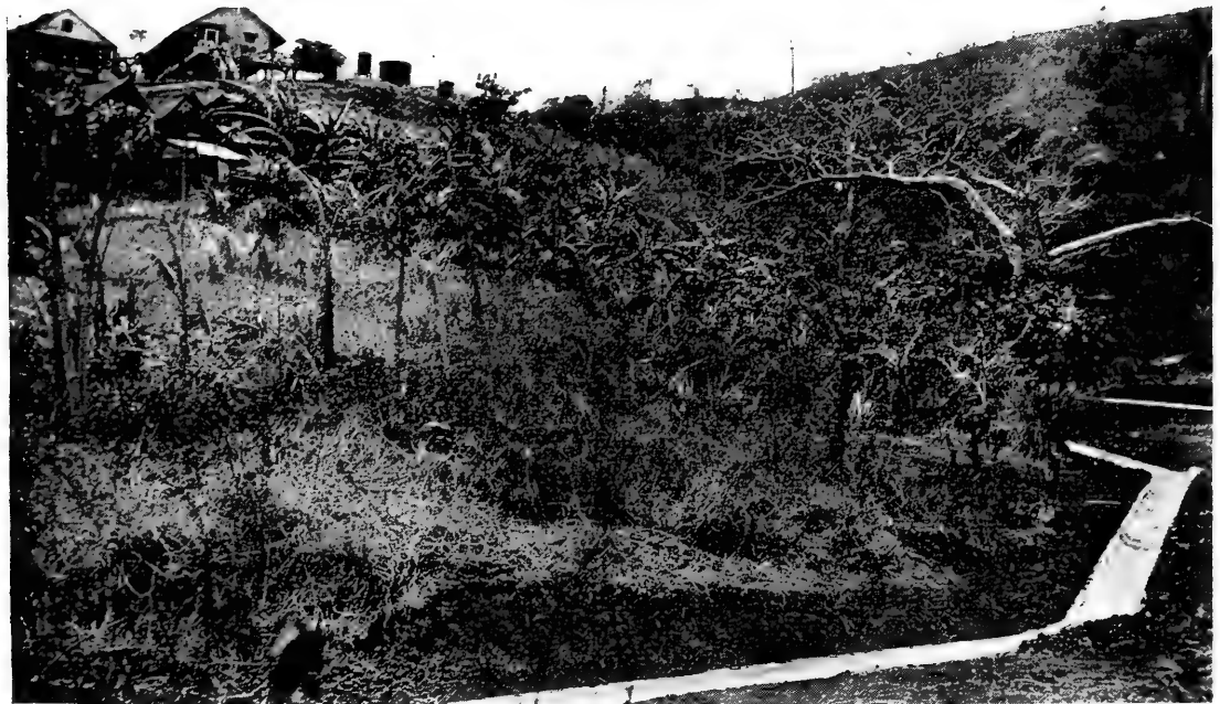
Concrete-lined ditch at Balboa
