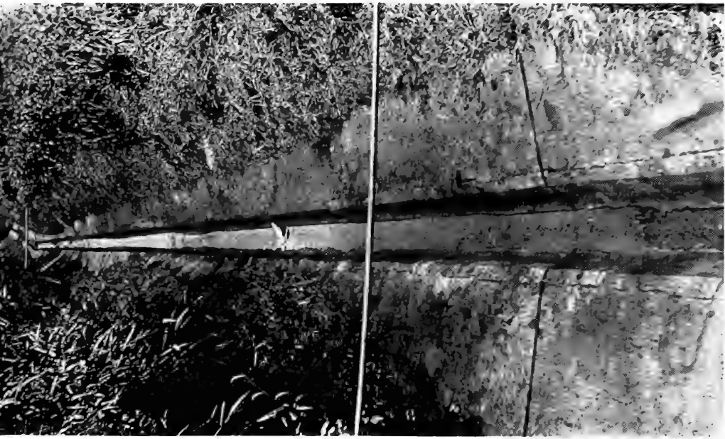
Concrete lining of a ditch of small cross-section
