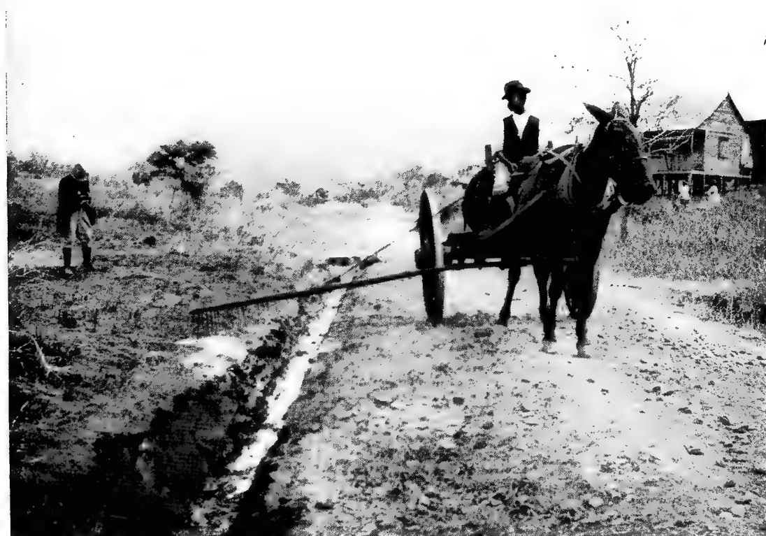
Oil cart for applying oil to roadside ditches
