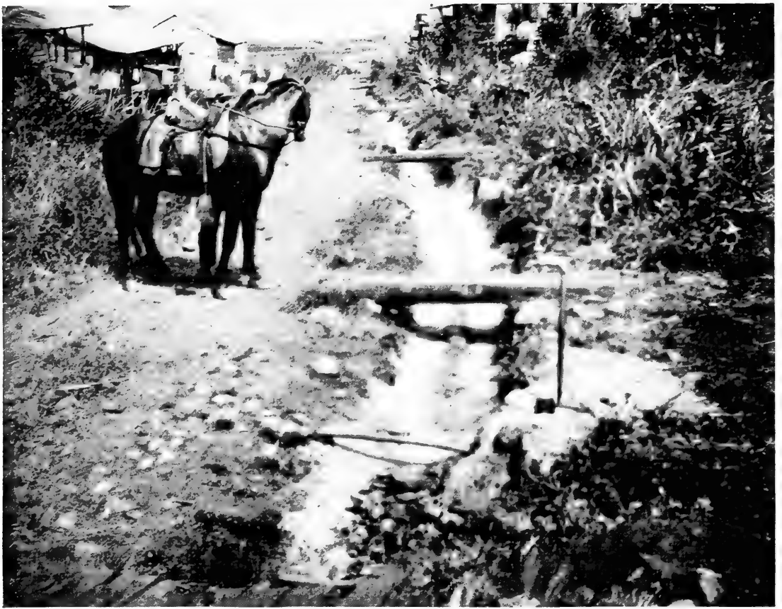
Concrete ditch lining
