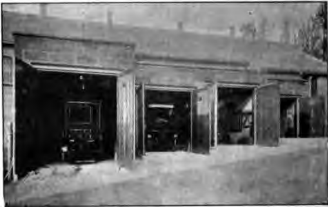
Fig. 3.—The Motor-houses at Broomhill, Tunbridge Wells
