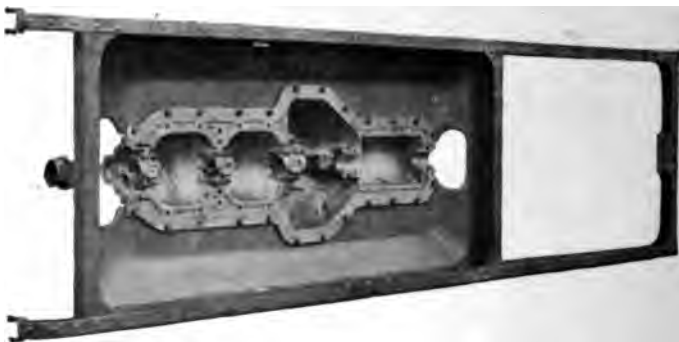
Fig. 2.—The Darracq Pressed Steel Frame
