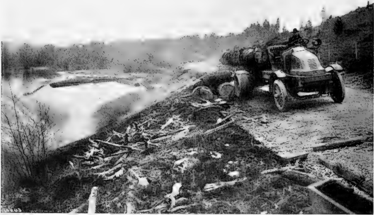
Unloading truck and trailer through the use of an incline, showing brow-skids and roll-way.
