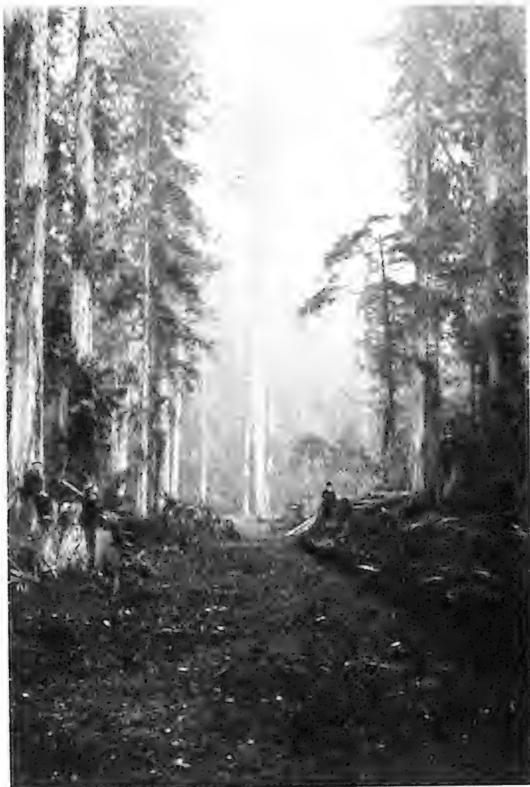
Sub-grade for motor truck logging road.
