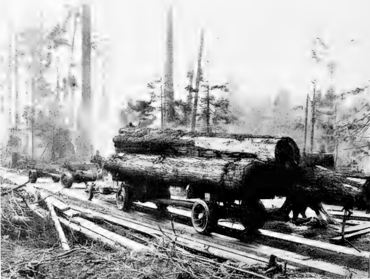
Turn-out on fore-and-aft plank road.
