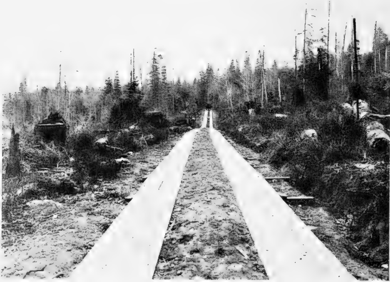
Fore-and-aft plank road with wedges on cross ties to facilitate the re-aligning of the planks.
