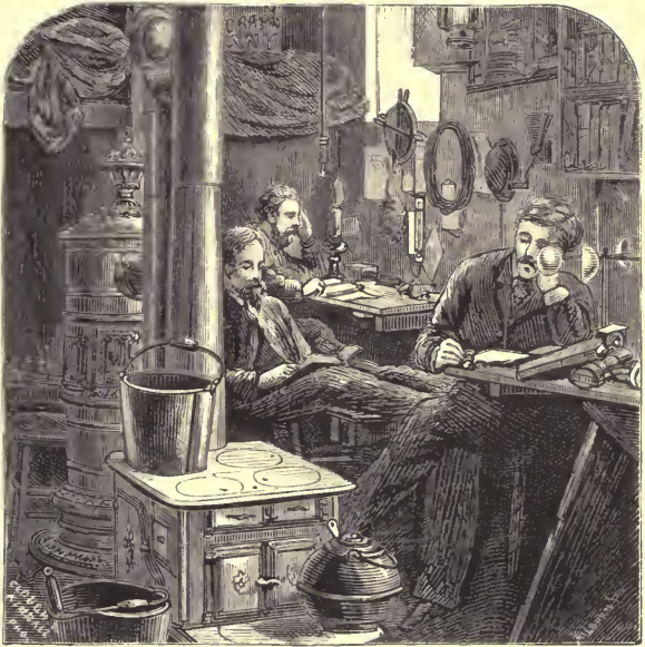
VIEW OF INTERIOR OF THE OBSERVATORY
