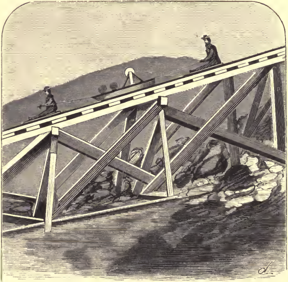
LAYING THE CABLE ON JACOB'S LADDER.
