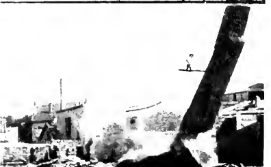
Result of the collision with the chimney.
