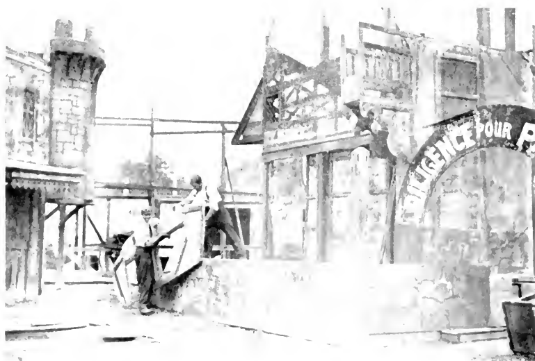
BUILDING A SOLID SET FOR "THE TWO ORPHANS."
