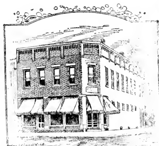
This is the Ribelin building, now occupied by Johnson Super Market
