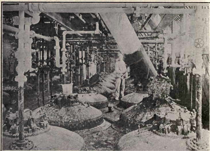
FIG. 151.—CHUTES TO DIGESTERS AT GARBAGE PLANT, NEW YORK.
