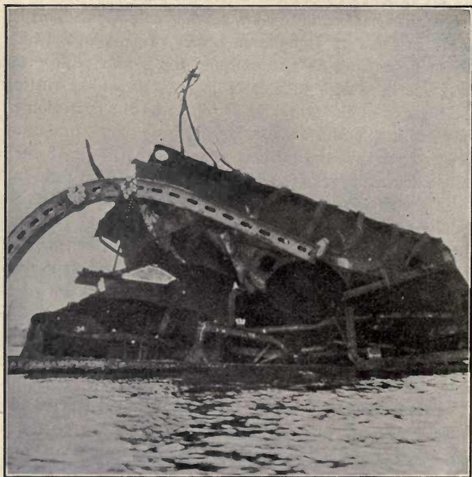
FIG. 229.—U. S. BATTLESHIP MAINE , HAVANA HARBOR. EXPOSED STEEL ABOVE WATER.
