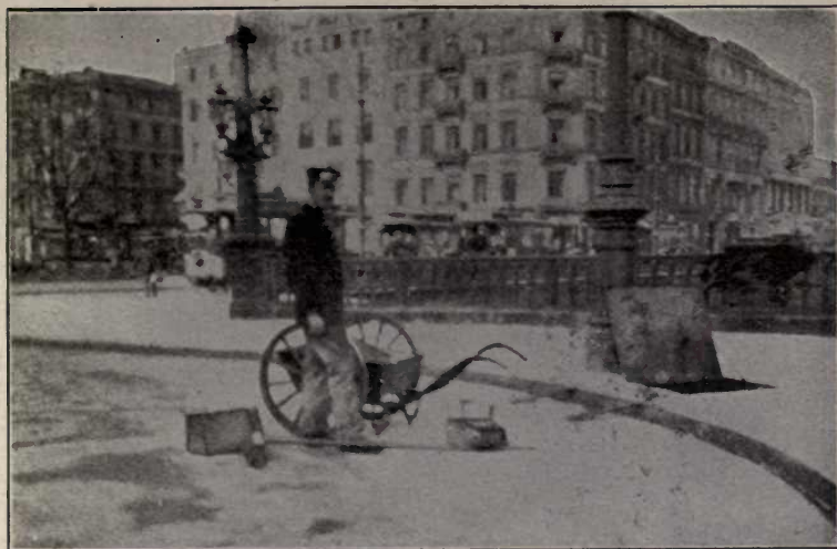
FIG. 127.—HAMBURG, GERMANY. STREET CLEANER WITH HIS APPARATUS ABOUT TO EMPTY A HANDCART FULL OF STREET SWEEPINGS INTO A TEMPORARY STORAGE PIT BENEATH THE SIDEWALK. (Courtesy of Dr. Soper.)
