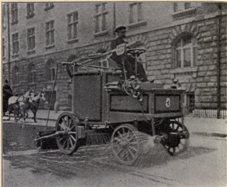
FIG. 144.—ELECTRICALLY DRIVEN MACHINE USED IN BERLIN, GERMANY, FOR CLEANING STREETS. (Courtesy of Dr. Soper.)
