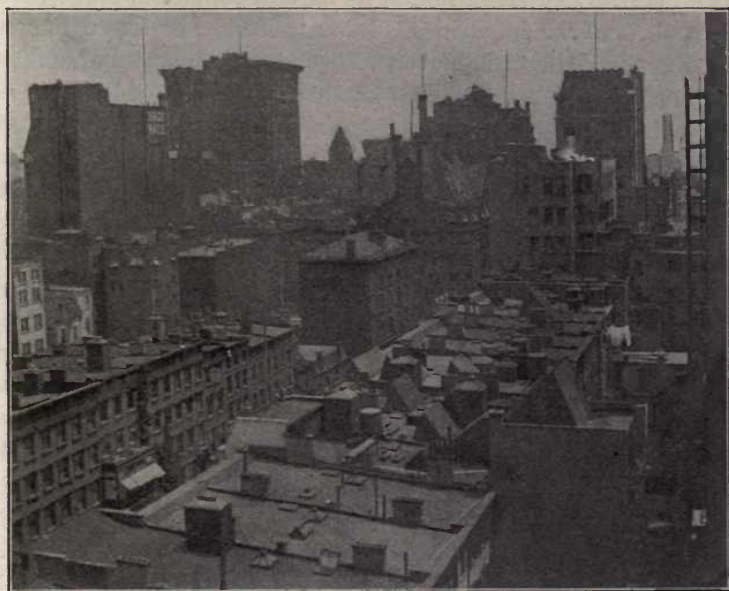
FIG. 194.—ANOTHER VIEW OF NEW YORK ROOFS.
