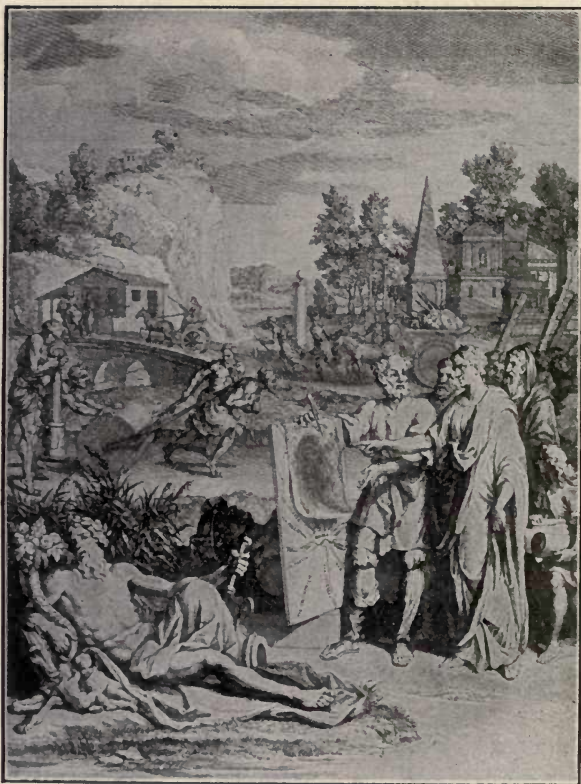
FIG. 105.—THE APPIAN WAY. OLD FRENCH ALLEGORICAL ENGRAVING SHOWING CONSTRUCTION IN PROGRESS.
