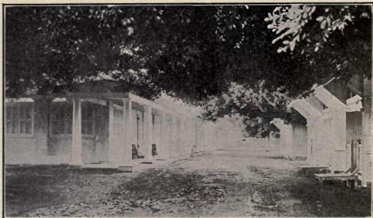
FIG. 235.—CONCRETE HOSPITALS BUILT IN CUBA OF LE BLANC CEMENT.
