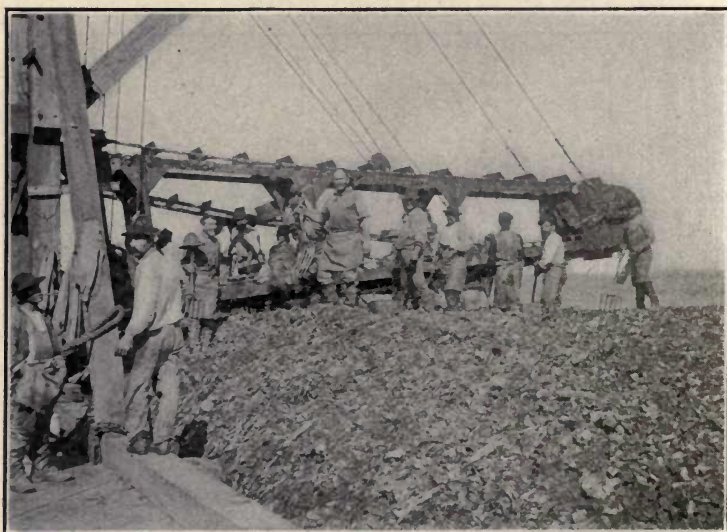
FIG. 157.—UNLOADING GARBAGE ON OUTBOARD CONVEYOR AT GARBAGE PLANT, NEW YORK.
