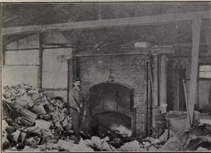
FIG. 167.—INCINERATOR IN COVERED DUMP IN BROOKLYN. TOP FEEDING. SMALLER ORIFICE IS BETTER.
