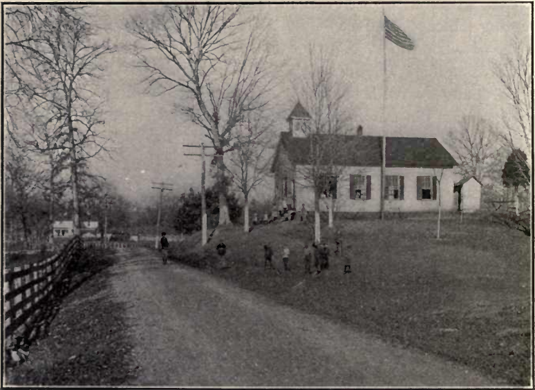
FIG. 111.—COUNTRY SCHOOL HOUSE ON GOOD ROAD NEAR KNOXVILLE, TENN.
