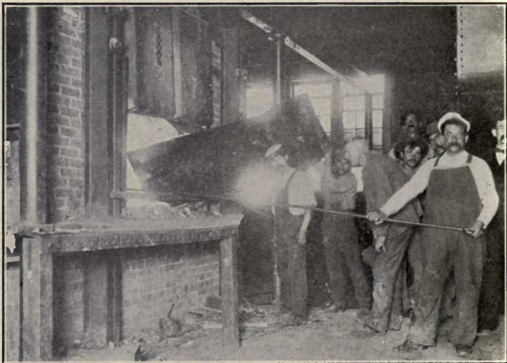
FIG. 166.—FEEDING AN OLD SOFA TO INCINERATOR. HEAT IS WASTED BY INTRODUCING SUCH LARGE OBJECTS.
