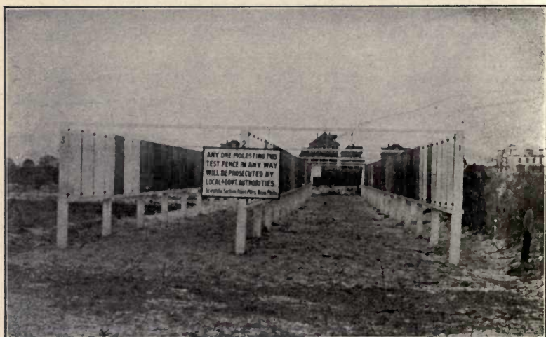
FIG. 228.—ATLANTIC CITY STEEL TEST PANELS.
