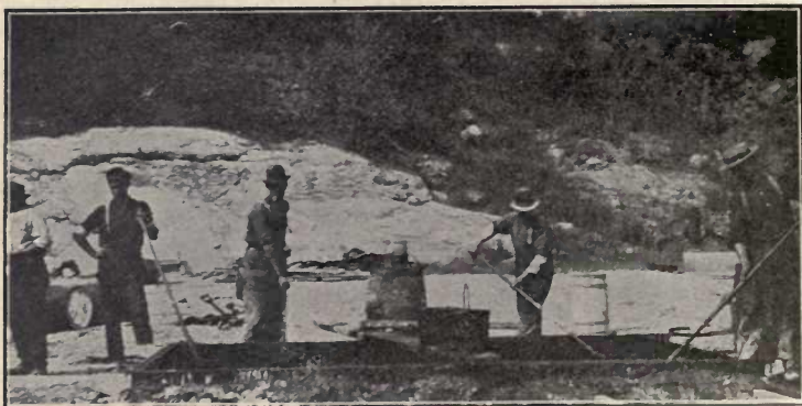
FIG. 116.—MIXING MATERIAL FOR "CANDY" ROAD, UTILIZING REFUSE FROM SUGAR REFINERIES.
