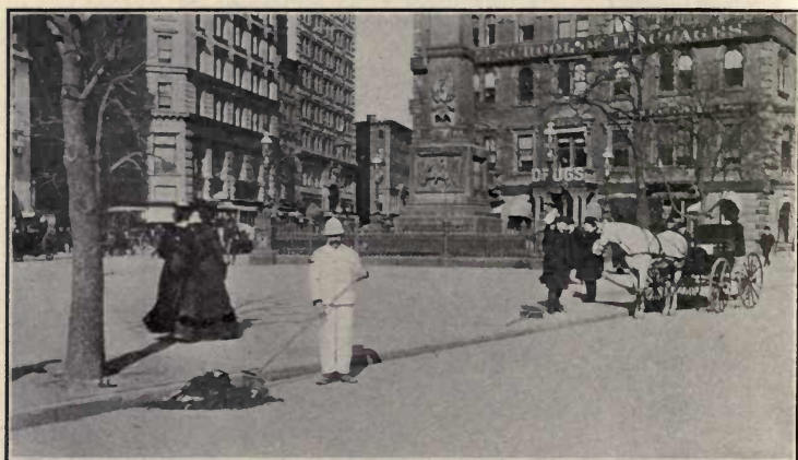
FIG. 121.—SWEEPER DEPOSITING SWEEPINGS IN GUTTER (OLD METHOD), NEW YORK CITY.
