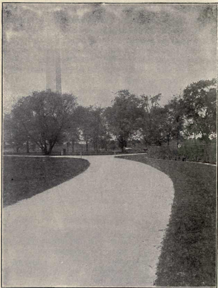
FIG. 115.—ROAD RECENTLY TREATED WITH CONCENTRATED WASTE SULPHITE LIQUOR IN AGRICULTURAL DEPARTMENT GROUNDS, WASHINGTON, D. C.
