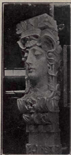
FIG. 234.—CASTING MADE OF WHITE CEMENT MORTAR.
