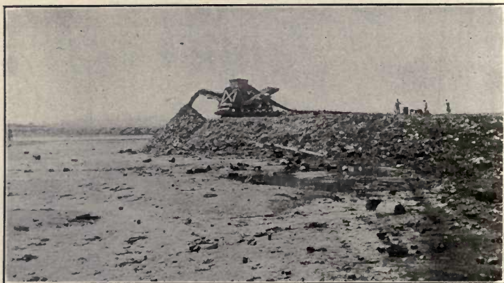
FIG. 161.—BELT CONVEYOR USED IN MAKING LAND WITH STREET REFUSE AT RIKER'S ISLAND, NEW YORK.
