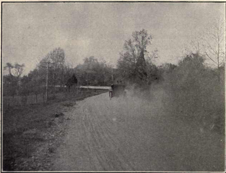
FIG. 112.—SHOWING DRIFT OF DUST TO ROADSIDE.
