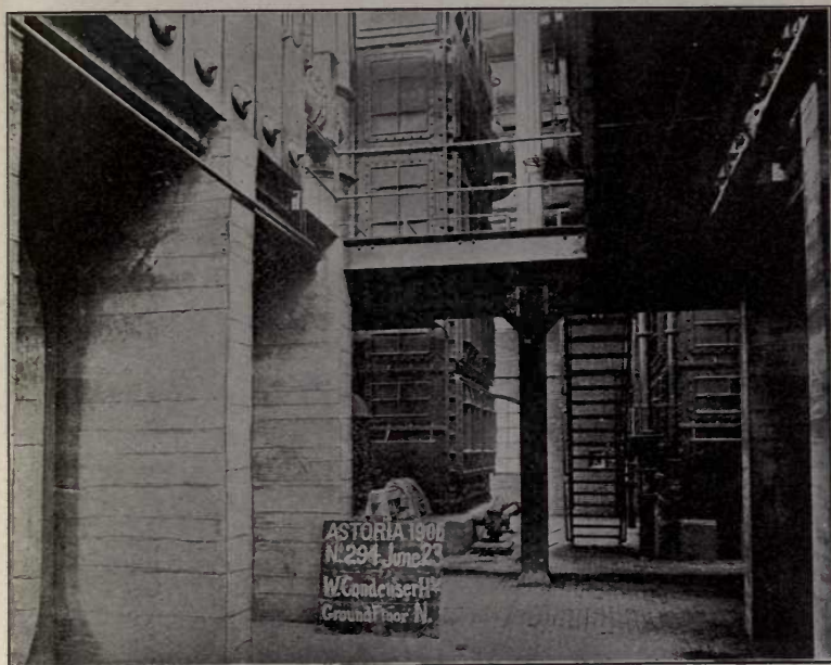
FIG. 178.—CONDENSERS, LOWER SECTION.
