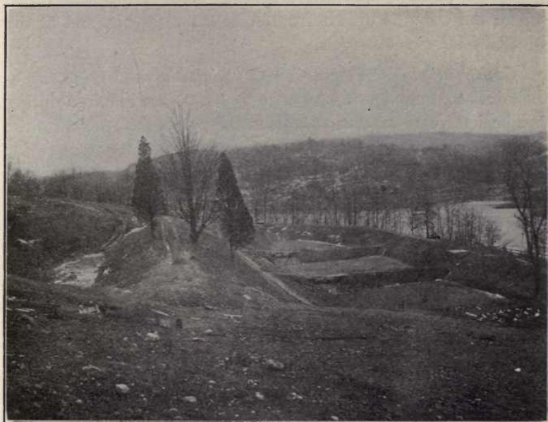
FIG. 30.—FILTER FOR CAMP AND TUNNEL DRAINAGE, CROTON DIVISION, CATSKILL AQUEDUCT.
