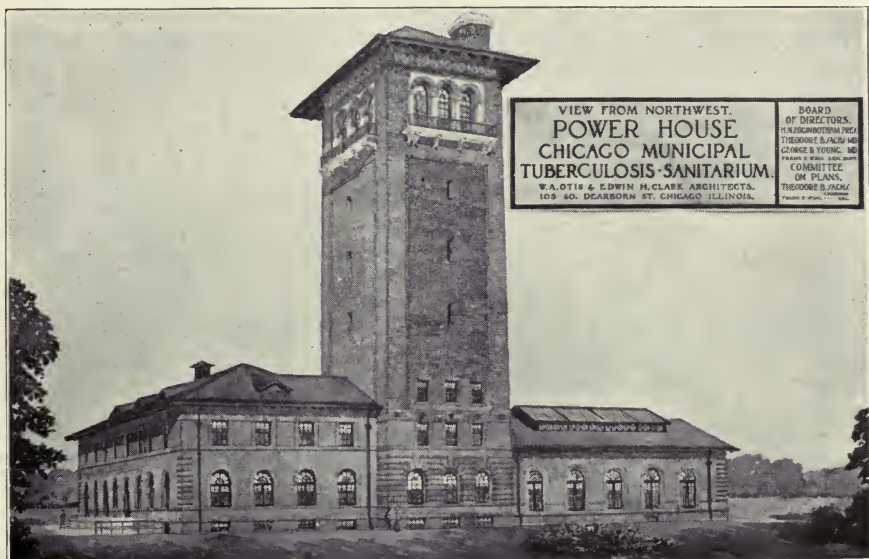
Power House and Laundry
