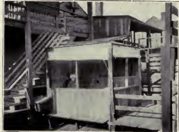
Shelter on a Roof
