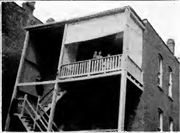
A Second Story Porch
