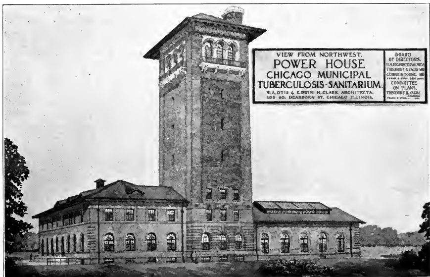
Power House and Laundry
