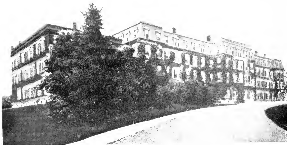
ABOVE—HIGH SCHOOL, HAVERHILL; BELOW, BRADFORD ACADEMY, HAVERHILL
