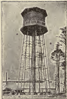
WATER TANK WITH STEEL TOWER
