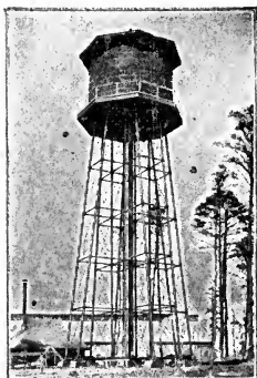
WATER TANK WITH STEEL TOWER
