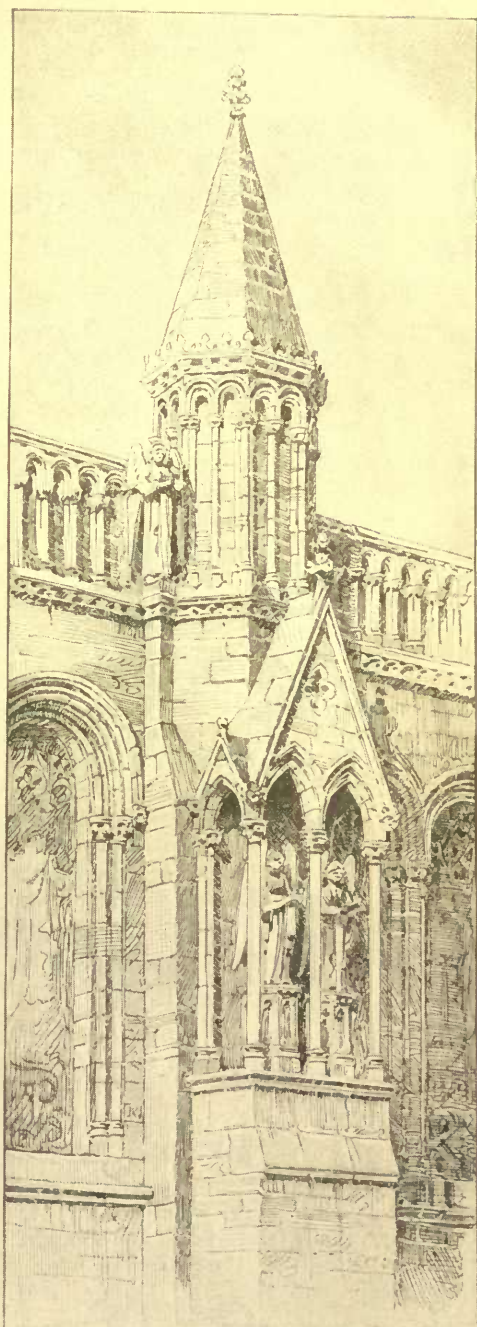
A STAIRCASE TURRET.
