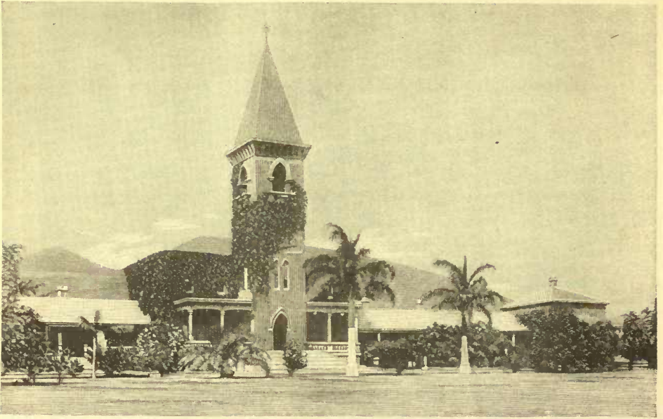
THE LUNALILO HOME FOR AGED HAWAIIANS, BUILT ACCORDING TO PLANS FOUND IN THE WILL OF THE YOUNG KING LUNALILO.
