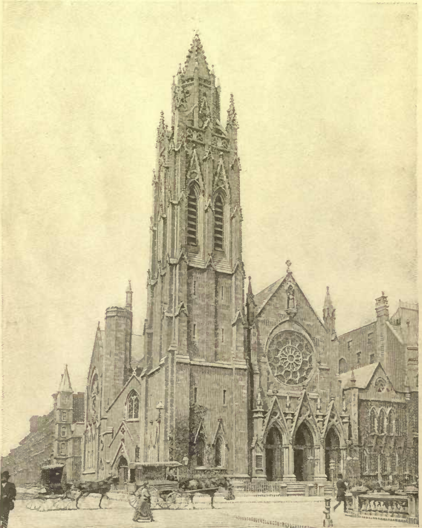
ST. THOMAS' CHURCH, FIFTH AVENUE AND FIFTY THIRD STREET.
