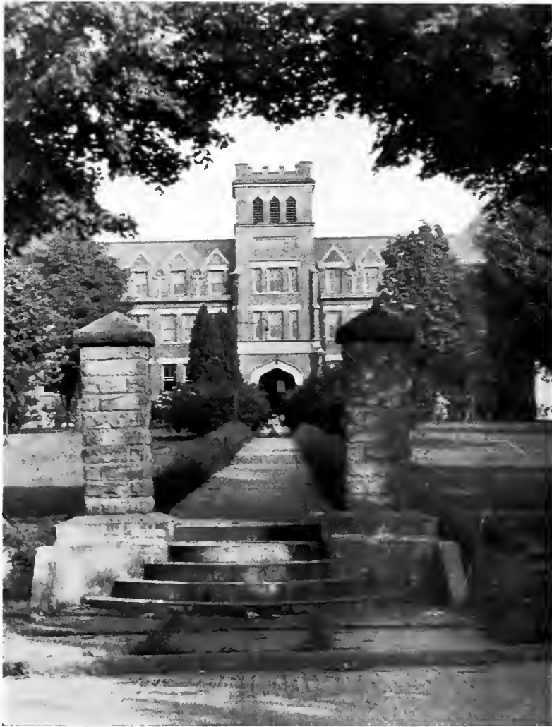
ADMINISTRATION BUILDING which contains the administrative offices, library, and the spacious Atkinson Chapel.
