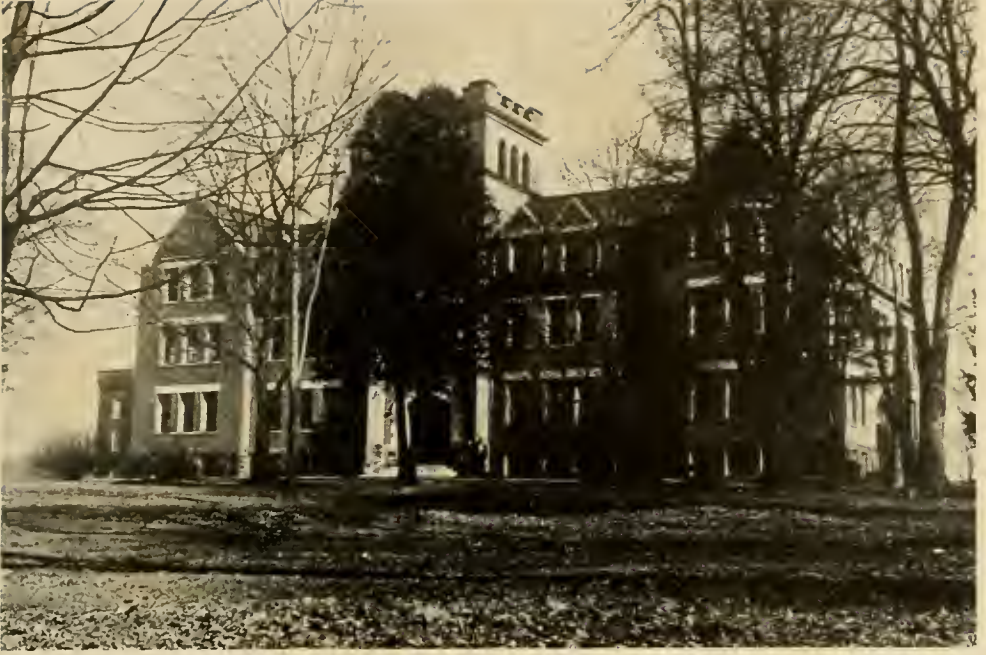
THE ADMINISTRATION BUILDING IS VIEWED FROM AN ANGLE
