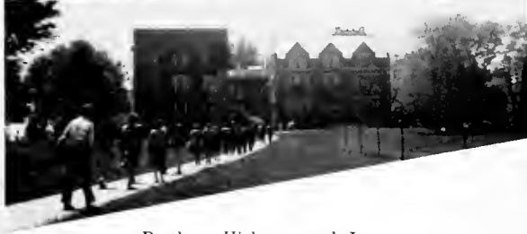
Brothers Hickman and Lang lay a board walk, while the students hit the trail to higher learning.
