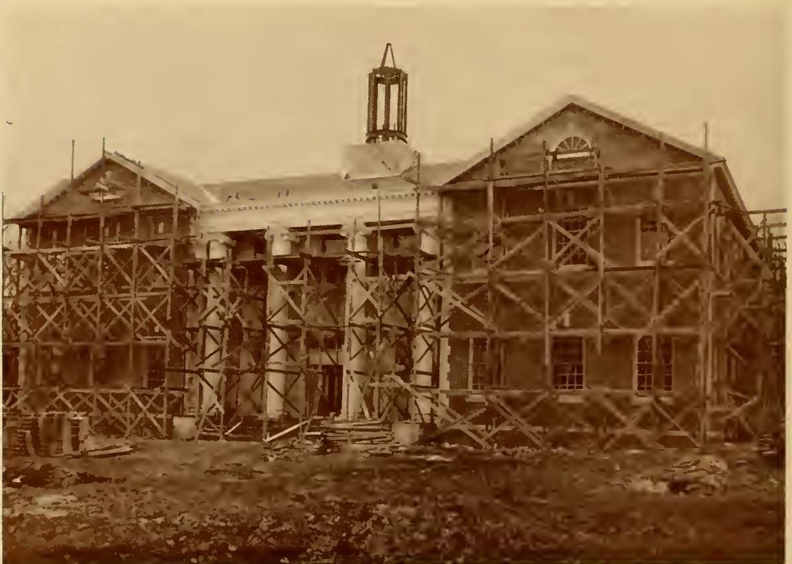
Building the Peiffer Memorial Library
