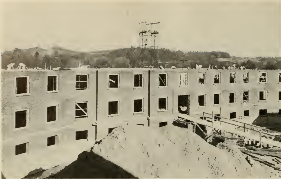
Construction on the third part of the men's quadrangle progresses.
