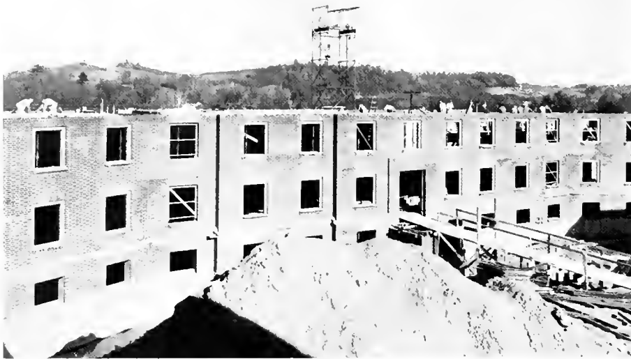
Construction on the third part of the men's quadrangle progresses.
