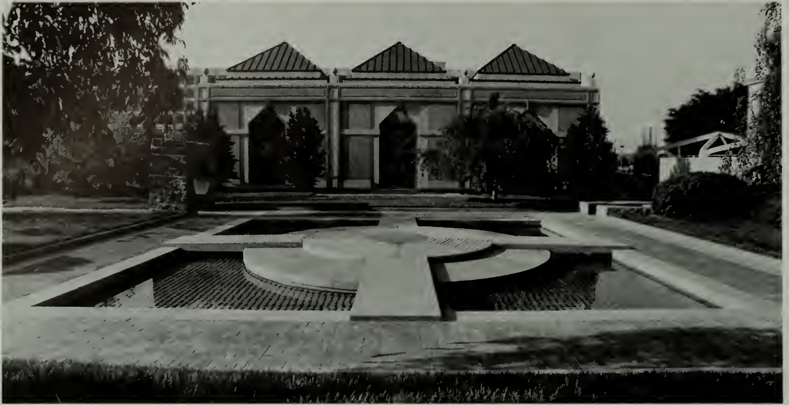
(a) The Entry Pavilion of the Arthur M. Sackler Gallery, Smithsonian Institution, Washington, D.C., is the gallery's only above-grade presence, with the bulk of its space—and its full architectural presence—not visible to the arriving visitor (Shepley Bulfinch Richardson and Abbott Architects, 1987). (b) In a complete reversal of tradition, the gallery's Central Staircase carries visitors down, not up, to its galleries, all of which are organized below-grade. (Courtesy Arthur M. Sackler Gallery. Photos: Kim Neilson)
