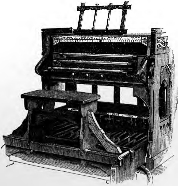
FIG. 9.—CONSOLE OF HOPE-JONES ELECTRIC ORGAN (With connecting Cable).
