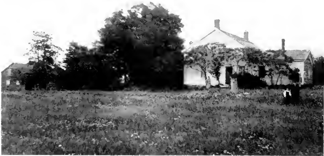
The Cross Homes, Richville, N. Y. Built in 1842 and 1852
