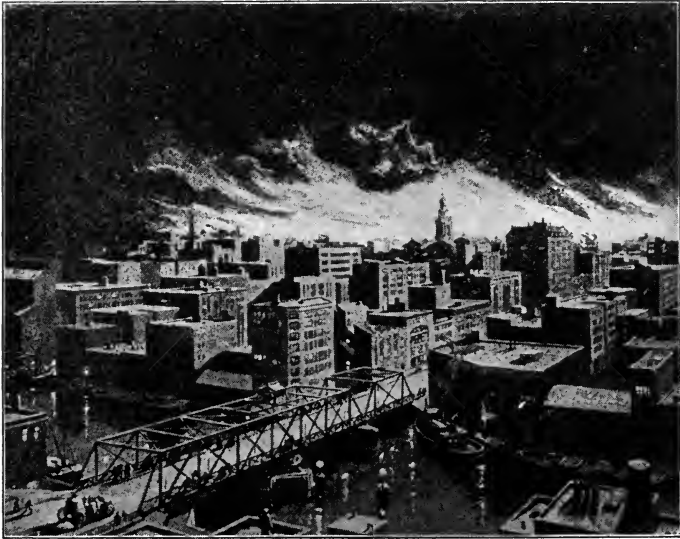
Somebody's Carelessness caused This Fire
